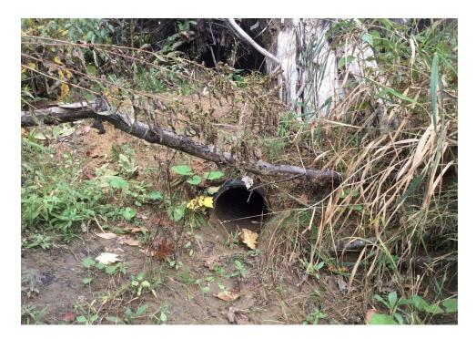
A properly installed cross drain culvert.
